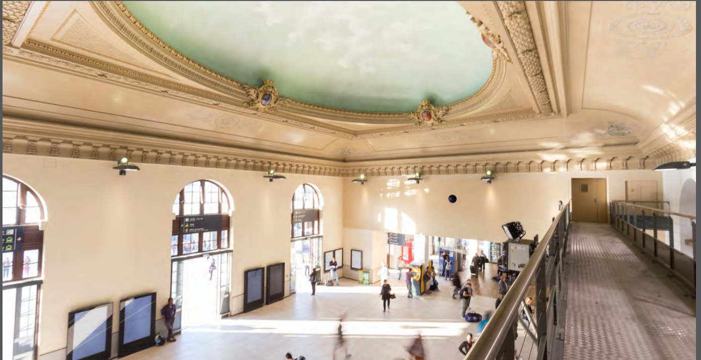
Nice train station - FRANCE - "Straw" colour acoustic walls - Installation: CLIBAT
